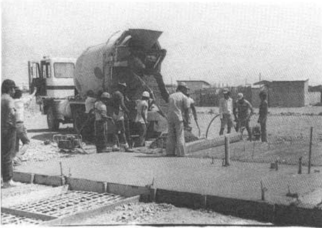
Fig. 15: The slab foundations, reinforced with bamboo cables and mesh and built 10 years ago, have no cracks
