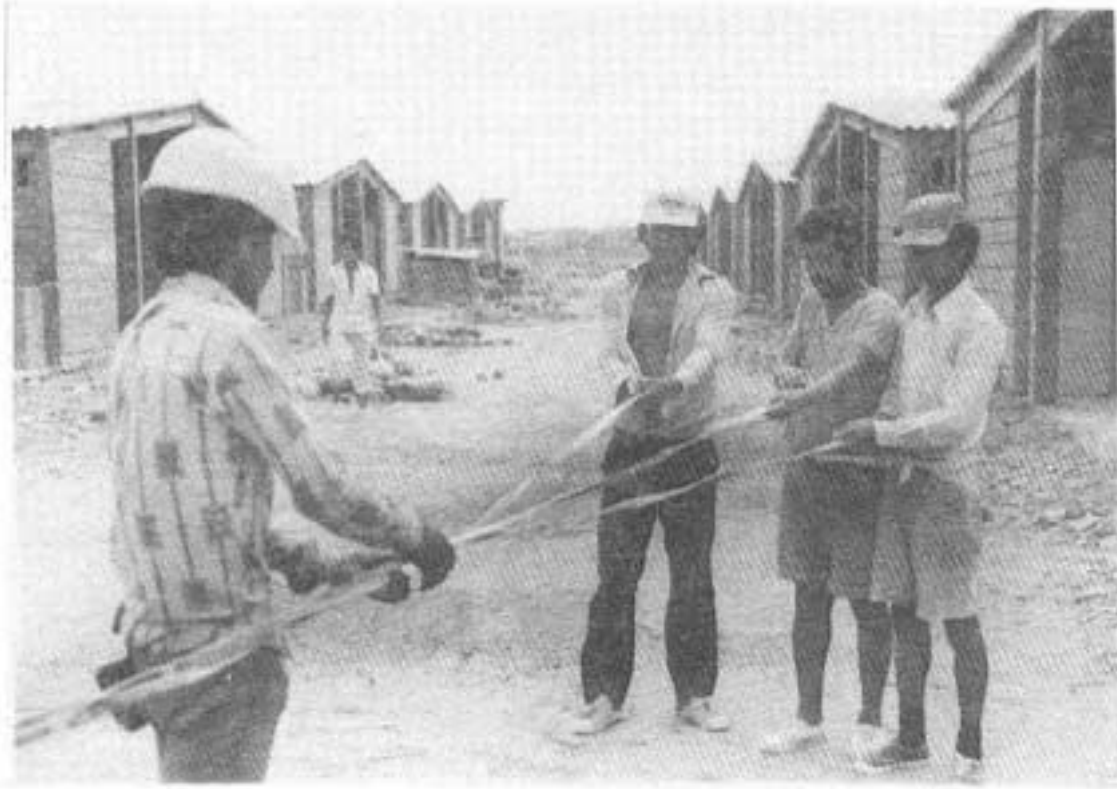
Fig. 8: Bamboo strands king twisted into cables
