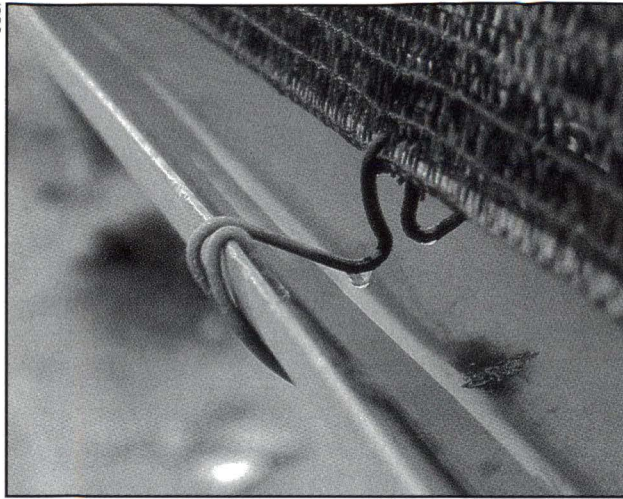
The water runs down the nets into gutters that drain into a 100,000-litre reservoir.
