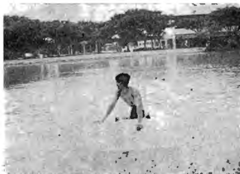
Fig. 11 Flotation test of a rectangular pontoon designed to serve as a floating pumping station.
