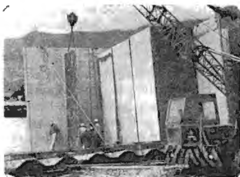
Fig. 10. Setting up pre-cast ferrocement elements of the caisson. Note projections of skeletal steel in panels, which ensure stronger joints. Joints are grouted after skeletal steel is welded in position.
