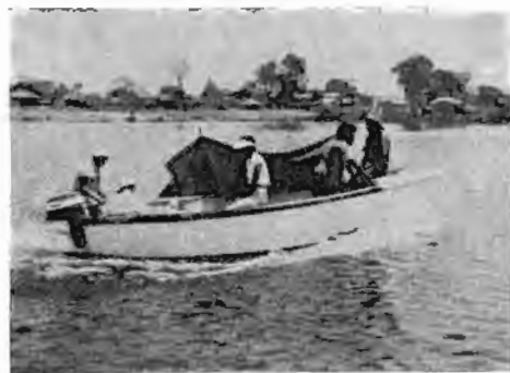
Fig. 6. 15-Foot ferrocement fishing launch produced on Lake Malawi.
