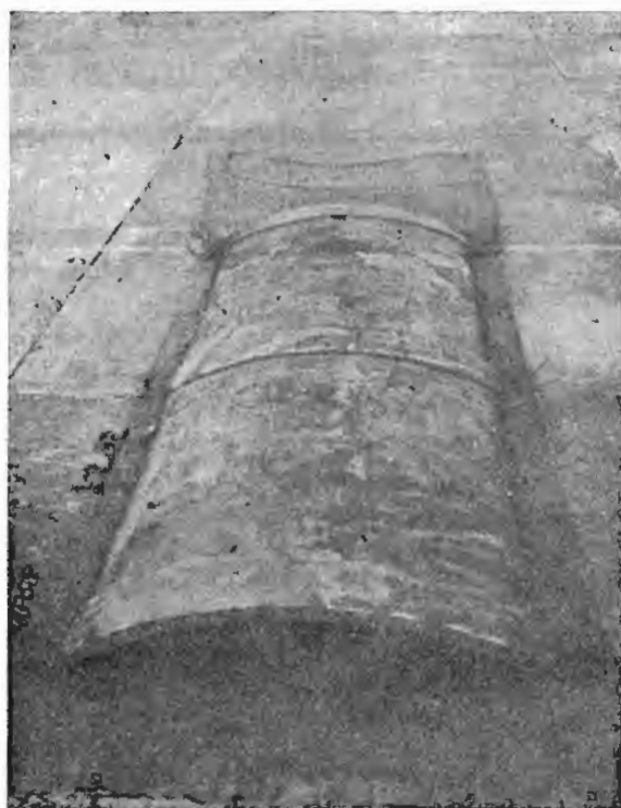
Fig. 1. Precast segmental unit with horizontal ribs. Note also mesh projections which facilitate construction of strong joints with similar other adjacent units.
