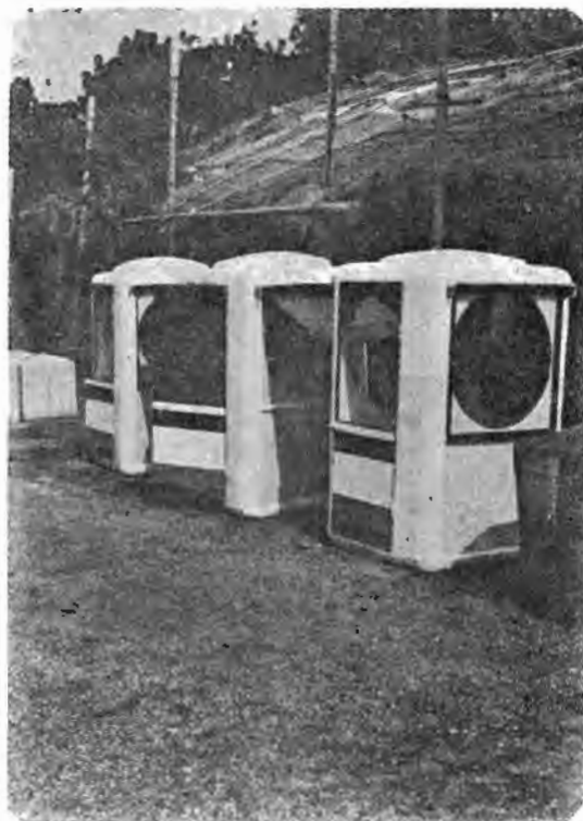
Fig. 20. Guard posts or mini kiosks made from ferrocement. Built-in steel frames for doors and windows make the design suitable for multipurpose use.
