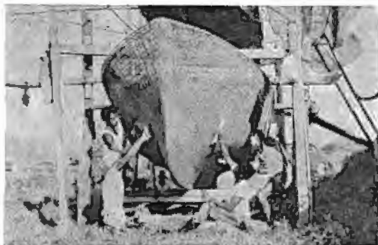
Fig. 25. A team of plasterers work on the hull under a temporary shed.
