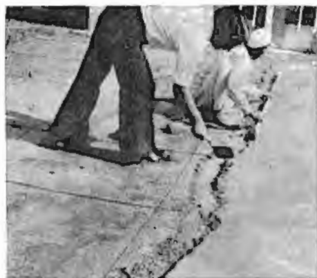
Fig. 8. If plastering cannot be finished within a day, the edge of a half-done job is tapered to improve adhesion with subsequent patch of mortar to be placed.
