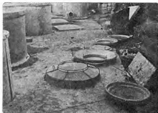
Fig. 12. Skeletal steel placed on masonry mould for the dome shaped roof unit. Photograph also shows lids for the roof and details of locking arrangement.
