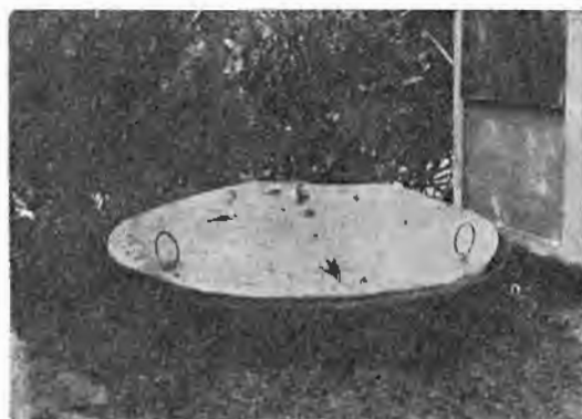
Fig. 19. A semi-underground biogas plant that is completely fabricated in ferrocement.
