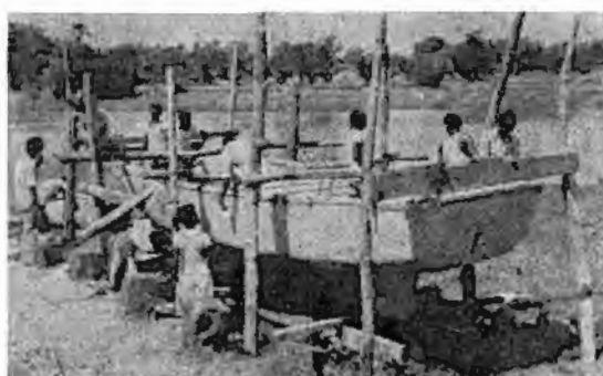
Fig. 26. Curing has been completed and minor finishing of the inside is undertaken.
