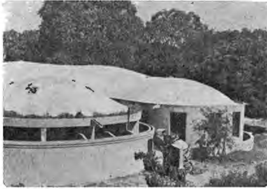
Fig. 5. A complex shell, W shaped in plan constructed at Ahmedabad. Interesting to note is the provision for ornamental plants along the edge beam.
