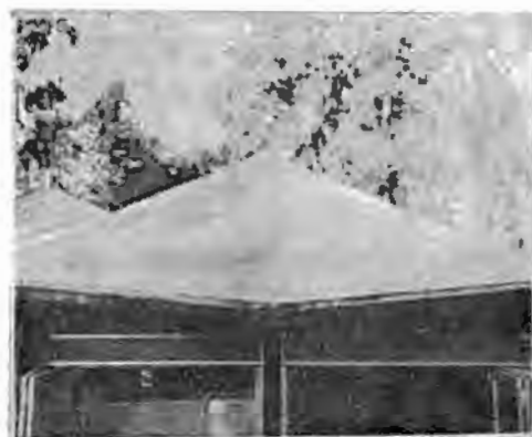
Fig. 17. Ferrocement waterproofing and protective layer over wooden roof, Ahmedabad, India.
