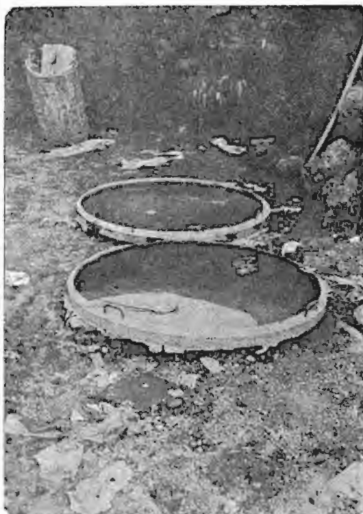
Fig. 11. Reinforced concrete base for the cylindrical units. Bases are provided with four lifting hooks to be used while handling the tanks and grain storage bins.
