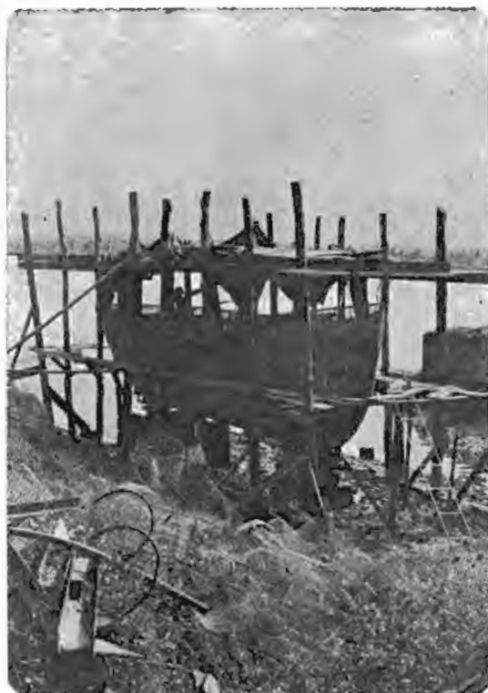
Fig. 13. 9.5 m hull is all meshed up and ready for plastering. Frames for the trawler were borrowed from a salvaged steel vessel.
