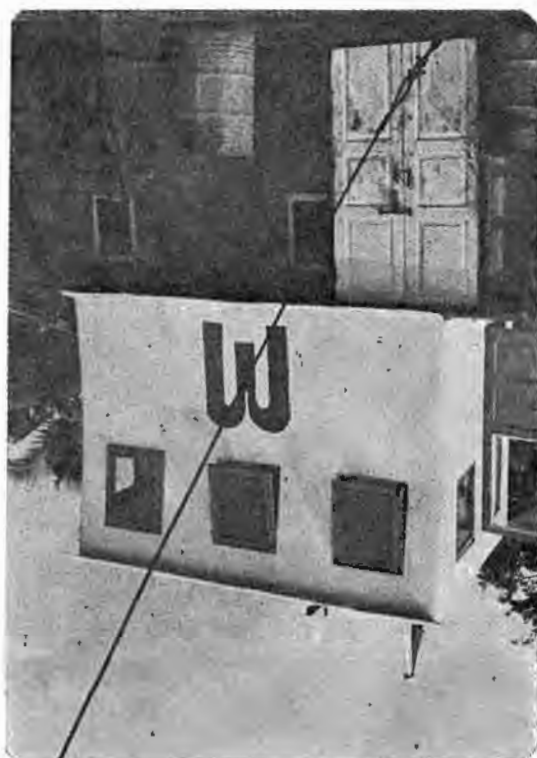
Fig. 15. Cabin and crew quarters fabricated in ferrocement (two storeyed) atop the deck of a steel salvage barge.
