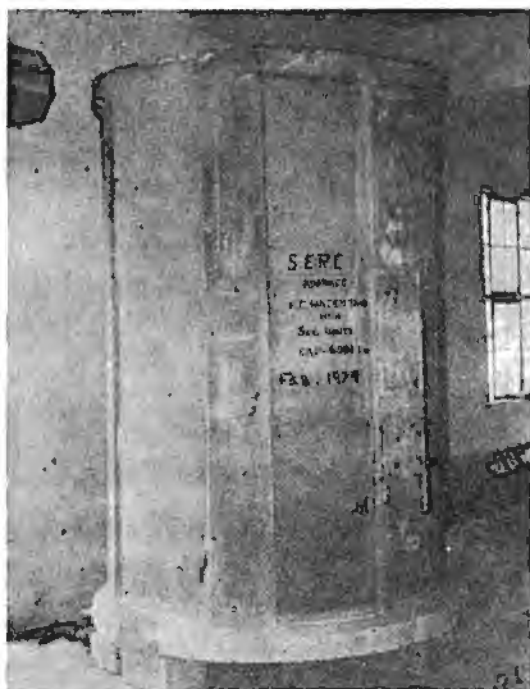
Fig. 3. A 6000 litre capacity tank made with ferrocement segmental units of 12 mm thickness. At joints vertical ribs of 25 mm are provided.
