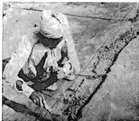
Fig. 7. Mortar is to be pushed under the wire-mesh layers using the lifting hook.
