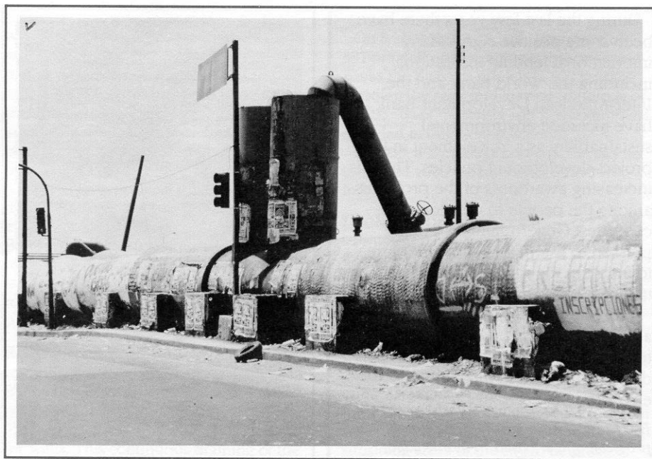
Aboveground pipe carrying drinking water in Mexico: subject to the abuse of the urban environment.
