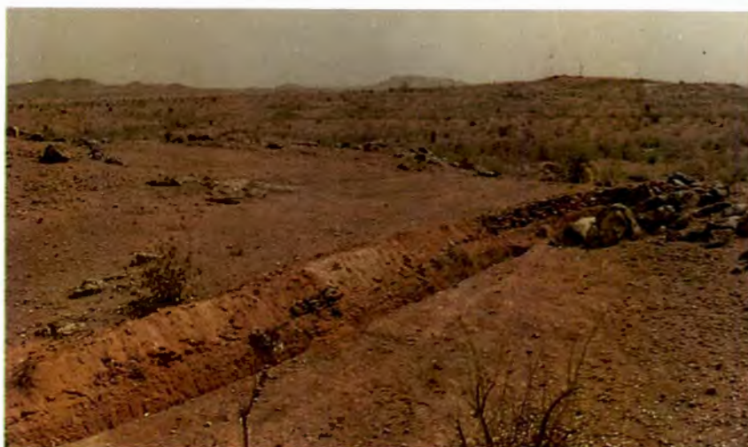
Cattle proof trench (left) and loose stone wall (extreme right) for protection against grazing
