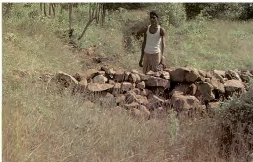
Loose stone gully plug to check the flow of rain water
