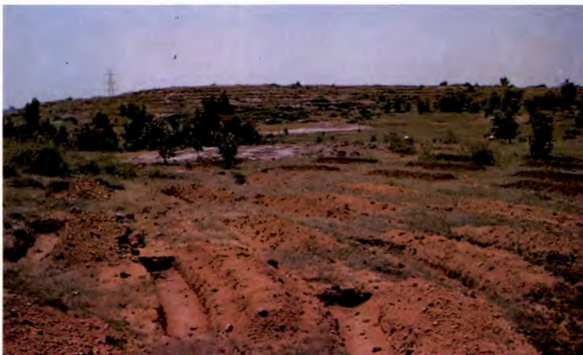
Contour trenches for checking run off and conserving soil and water
