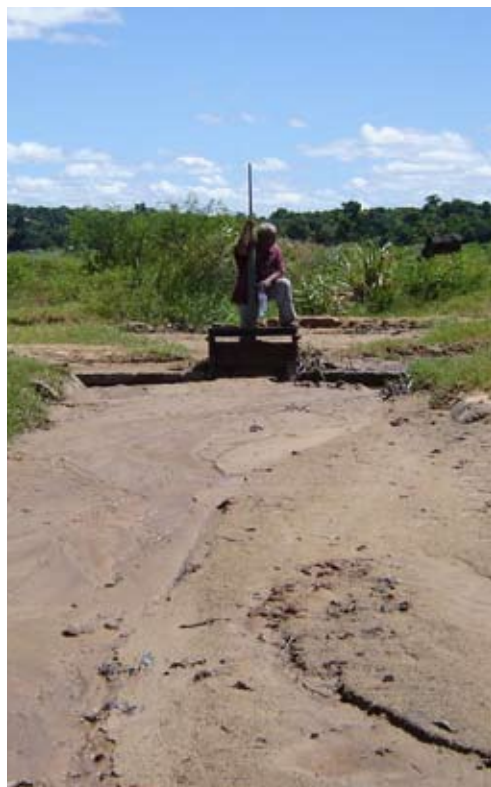
Gap and sand on the main canal called "Karambo" of the check dam of Amboromalandy (Photo : Nosy Alizany, CCAA-Madagascar)
