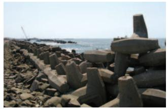
Hard adaptation measures such as this sea wall are expensive to build and need maintenance due to wave damage. *Photo: IDRC / Mohammed Yahia*
