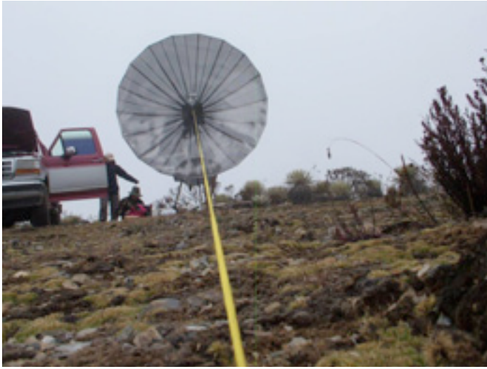
Figure 11.33: Aiming the antenna at el Águila.
