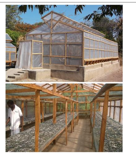
Fig. 1 Picture of the outside (upper) and inside (lower) view of a fish solar tent dryer
