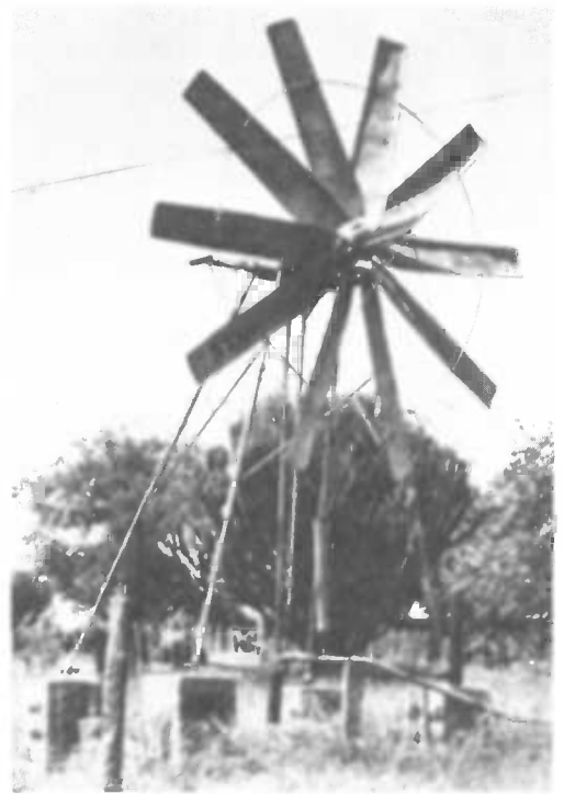
Fig. 5. Front view of a Mbita windmill with twisted blades.
