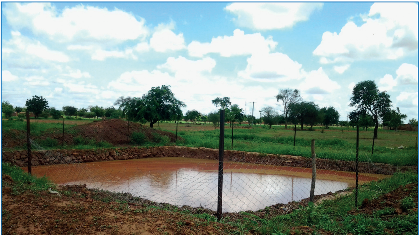
Runoff catch basin measuring 250 m 3 , built with local materials: lateritic bottom and stone-lined walls
