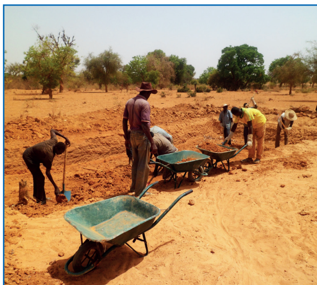
Construction of a runoff catch basin built with low-cost, local materials
