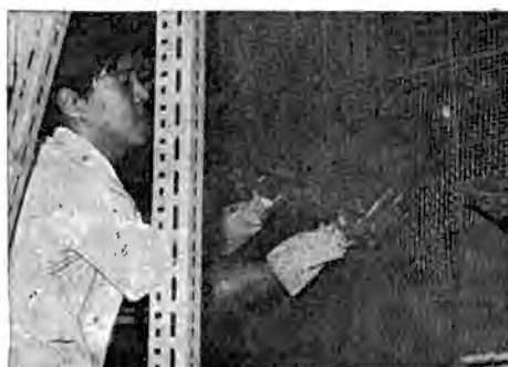
Fig. 6. Plastering of tank wall.
