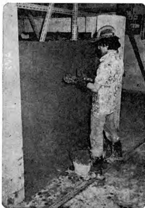
Fig. 14. Plastering of tank walls.
