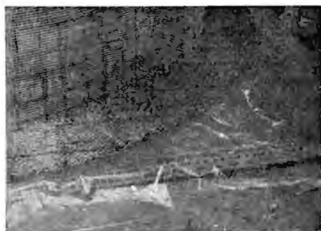
Fig. 5. Outside view of cylindrical wall and base plate after laying of wire mesh prior to plastering.
