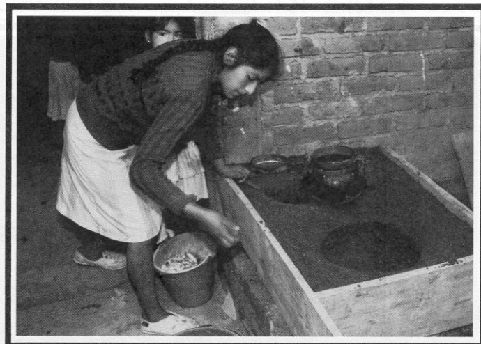
This modified "Lorena" stove under construction burns less than half the wood consumed by traditional means.
