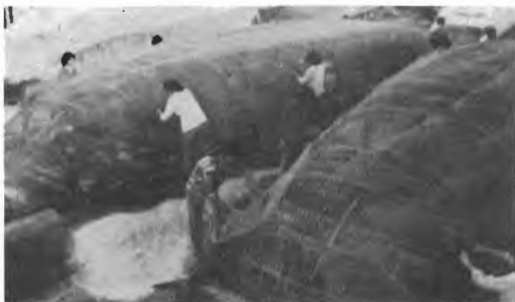
Placing the wire mesh over the ferrocement armature.
