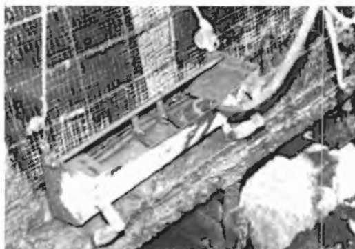
Close-up of the high frequency grouting equipment from the hanging trolley.
