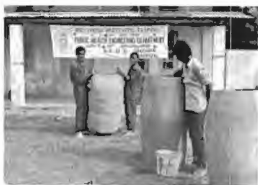
Casting of ferrocement water jar during training-cum-demonstration course at Dimapur (Nagaland), October 1988.
