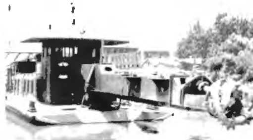
Fig. 42. A 168 m, 80 m 3 /hr output and 10 km/hr suction cutter dredger operating in Xiaoqing River, Jinan City.
