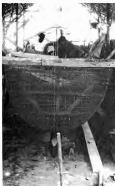
Fig. 2. The completed armature.
