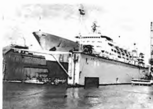
A 5000 t ferrocement floating dock.
