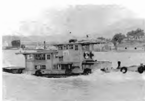
Fig. 29. "Ronggangtuo No. 203," a 15.4 m, 120 hp harbor tug. Built in 1958, it is the first ferrocement harbor tug used in China and has been in operation in Fuzhou Port since then. Compared with wooden hull, the savings in repair cost for the ferrocement hull amounts to a sum enough to build another two similar tugs.
