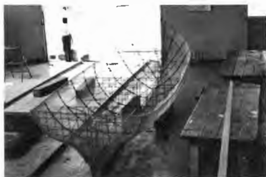
Fig. 2. The completed armature.
