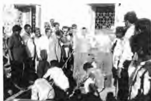
Demonstration of the casting of ferrocement water tank by skeletal cage system during training-cum-demonstration course at Gulbarga (Karnataka) in December 1988.
