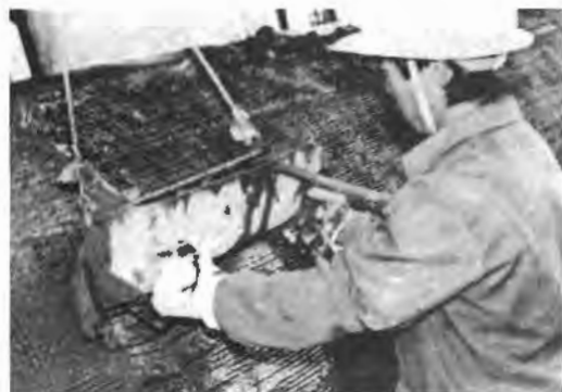
Plastering the cement mortar by high frequency equipment.
