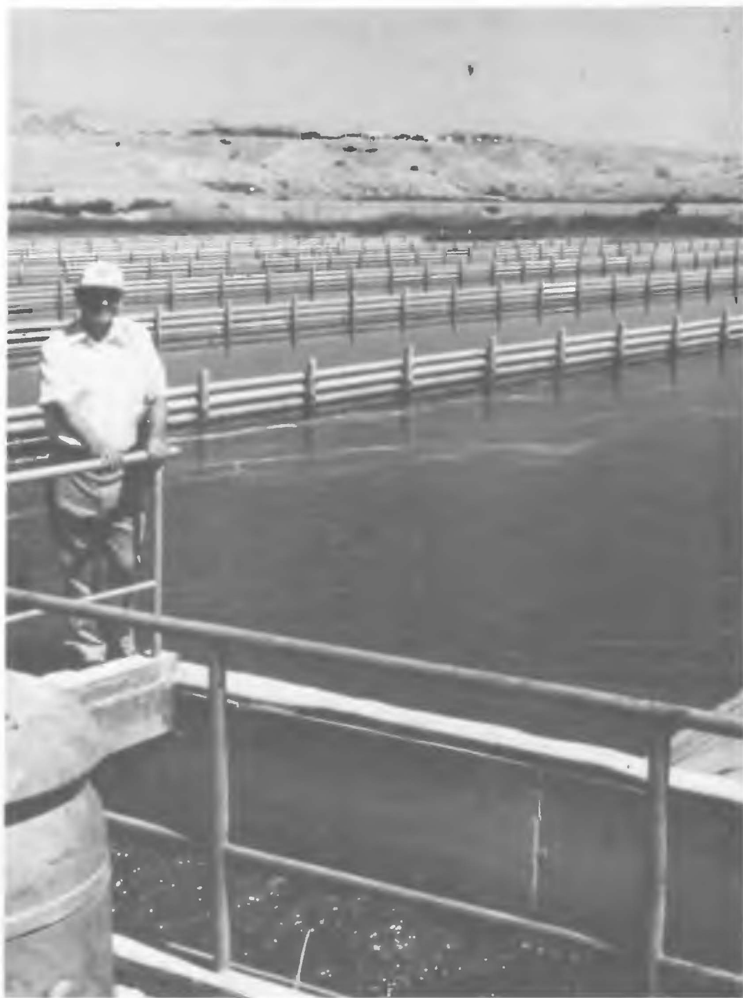
The full-scale high-rate algae ponds used to treat domestic wastewater at Eilat, Israel (courtesy G. Shelef).
