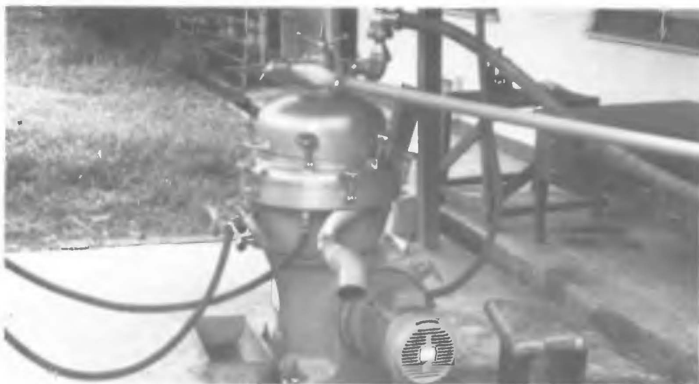
The pilot-scale centrifuge used to dewater the algal floc (courtesy Primary Production Department, Singapore).
