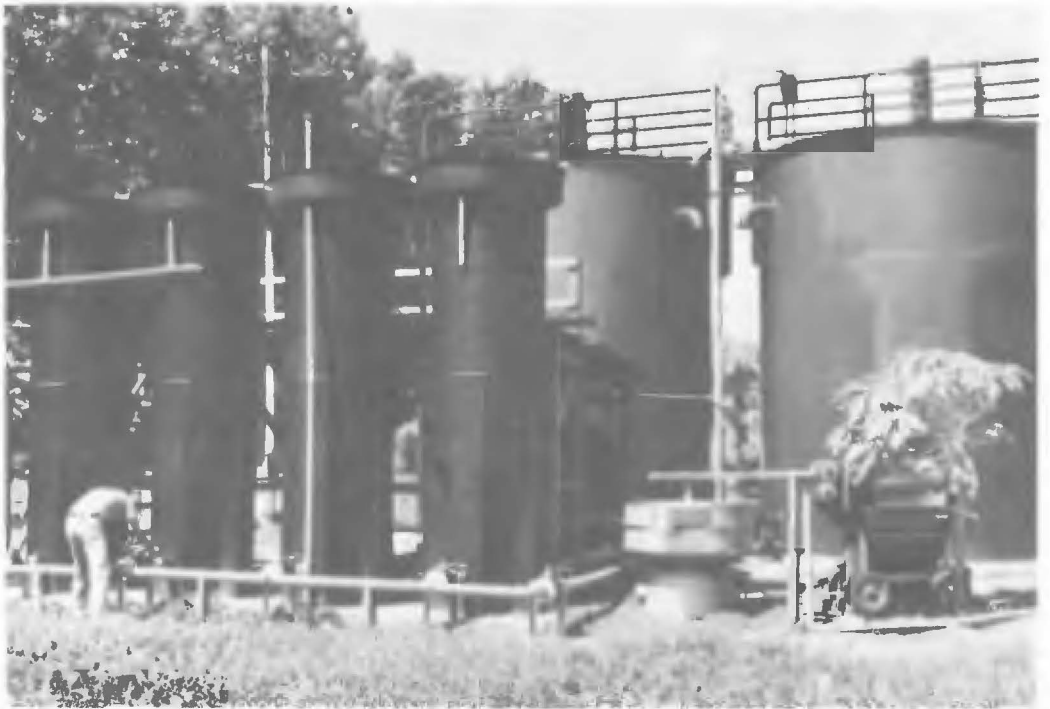
The storage tanks (in background) and the primary clarifiers used for pretreatment of wastewater fed into the high-rate algae ponds.
