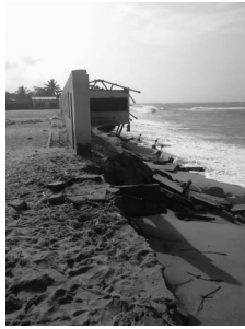
Figure 4. Collapsed school building in Fuvemeh community, which illustrates the effect of coastal erosion on vulnerable delta communities (taken June 2016).
