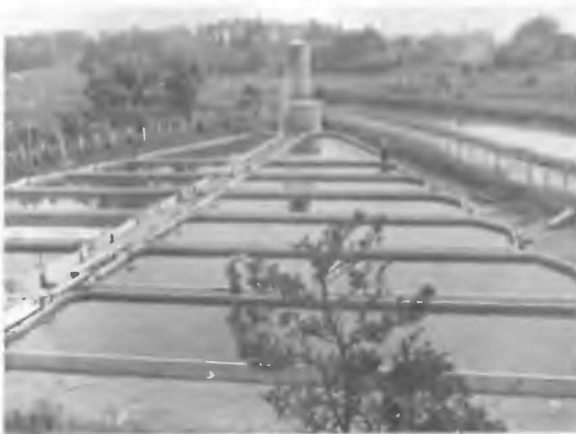
Fig. 18. Series of small concrete ponds which can be adopted for the rearing of larval fish.
