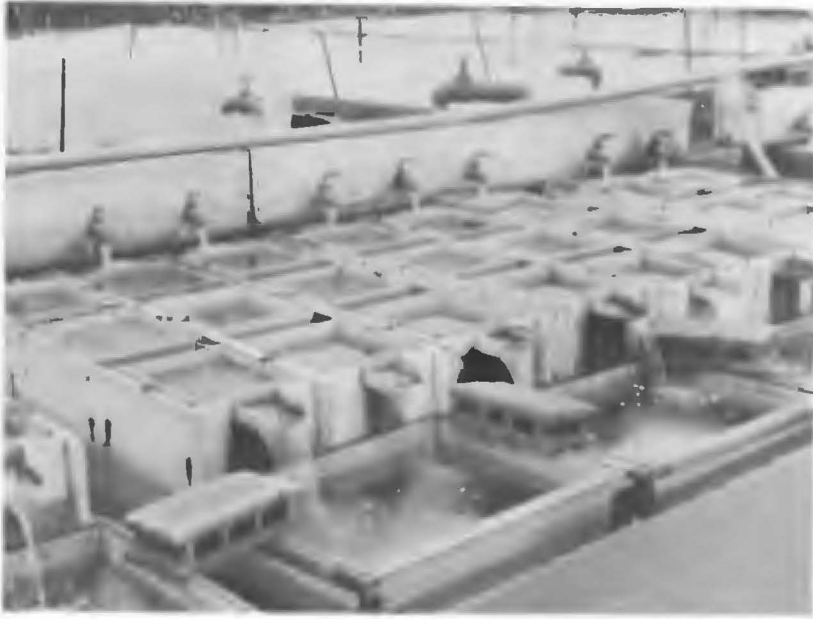
Fig. 17. Battery of hatching boxes in operation. Note one fry-receiving container connected to one pair of hatching boxes.
